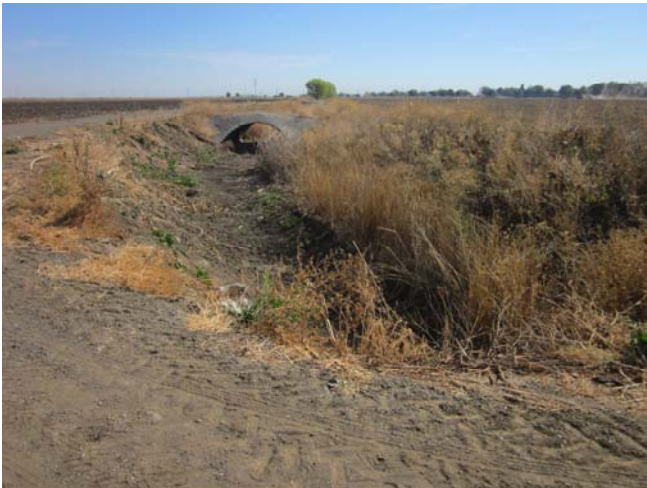
Photo 15. View east from the eastern edge of the MRIC site toward the Mace Drainage Channel (looking downstream) along the sewer line alternative. An open bottom arch crossing visible in distance. 7 October 2014.
