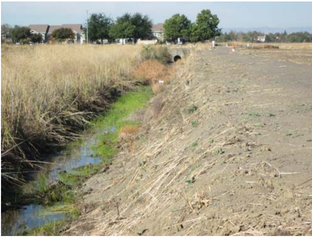
Photo 7. View west toward Mace Drainage Channel in western portion of the PSA. One of two culverts that pass water beneath Mace Blvd visible in distance. 7 October 2014.
